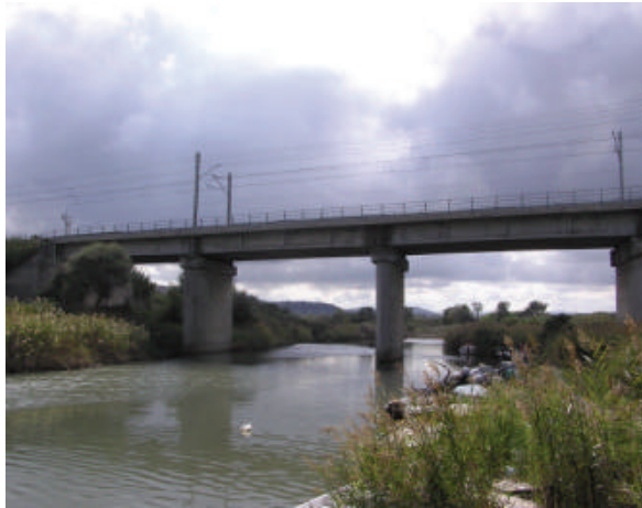
Fig. 1. Sinello railway bridge (Garibaldi et al., 2005).
